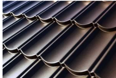
Zircon in roof tiles increase solar reflection and reduce heat
