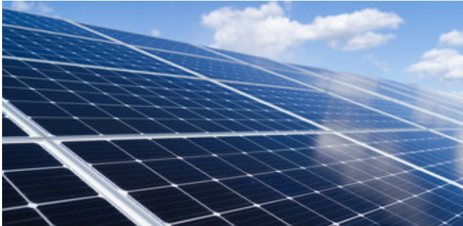
Construction of the solar farm began in mid-October
