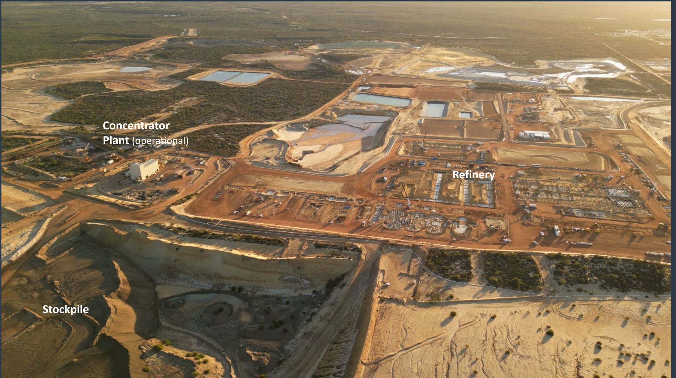
Eneabba rare earths refinery, Western Australia
