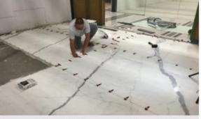
Large, thin, slab tiles can be 6mm thick
