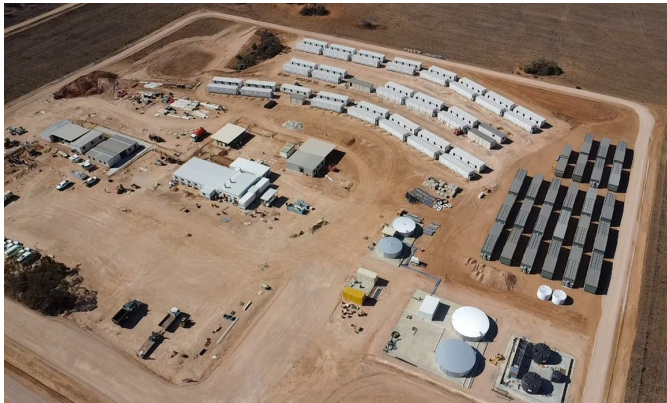
Early stages of Iluka's accommodation camp at the Balranald mine site
