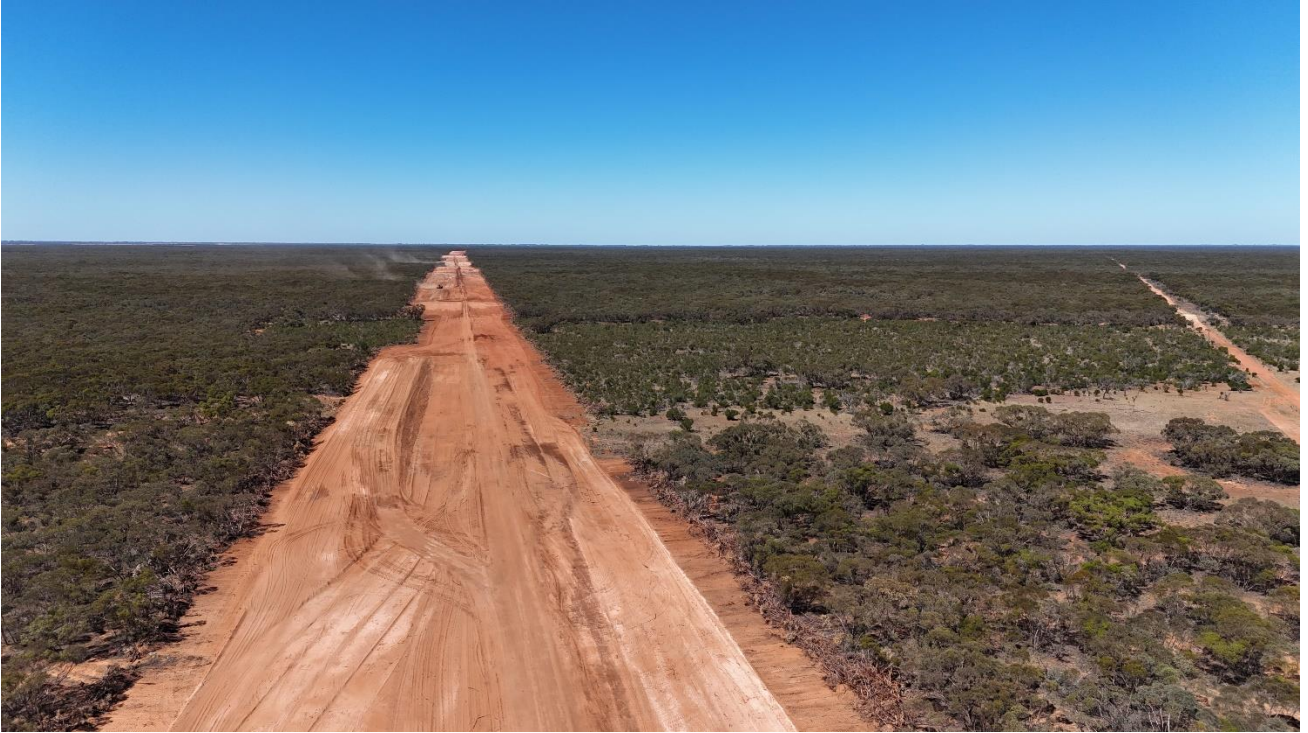
Mine access road clearing (March 2024)
