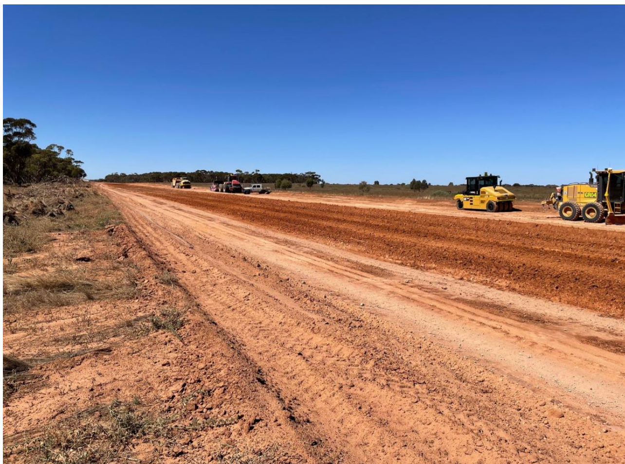
Photo 1: Construction of new site access road in 2024.
