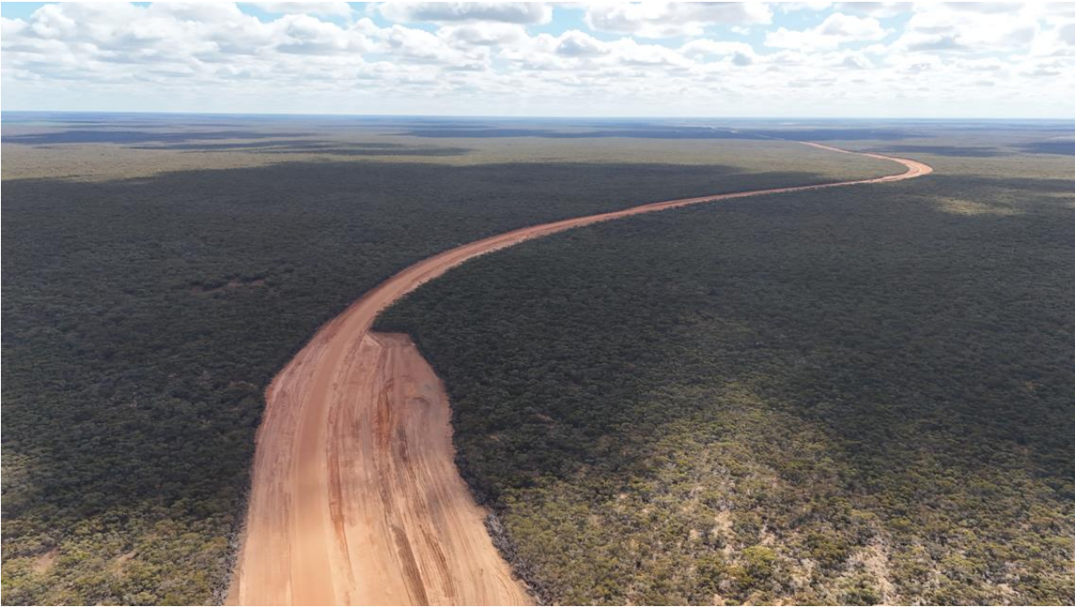
Photo 2: Aerial view of construction of new site access road in 2024.
