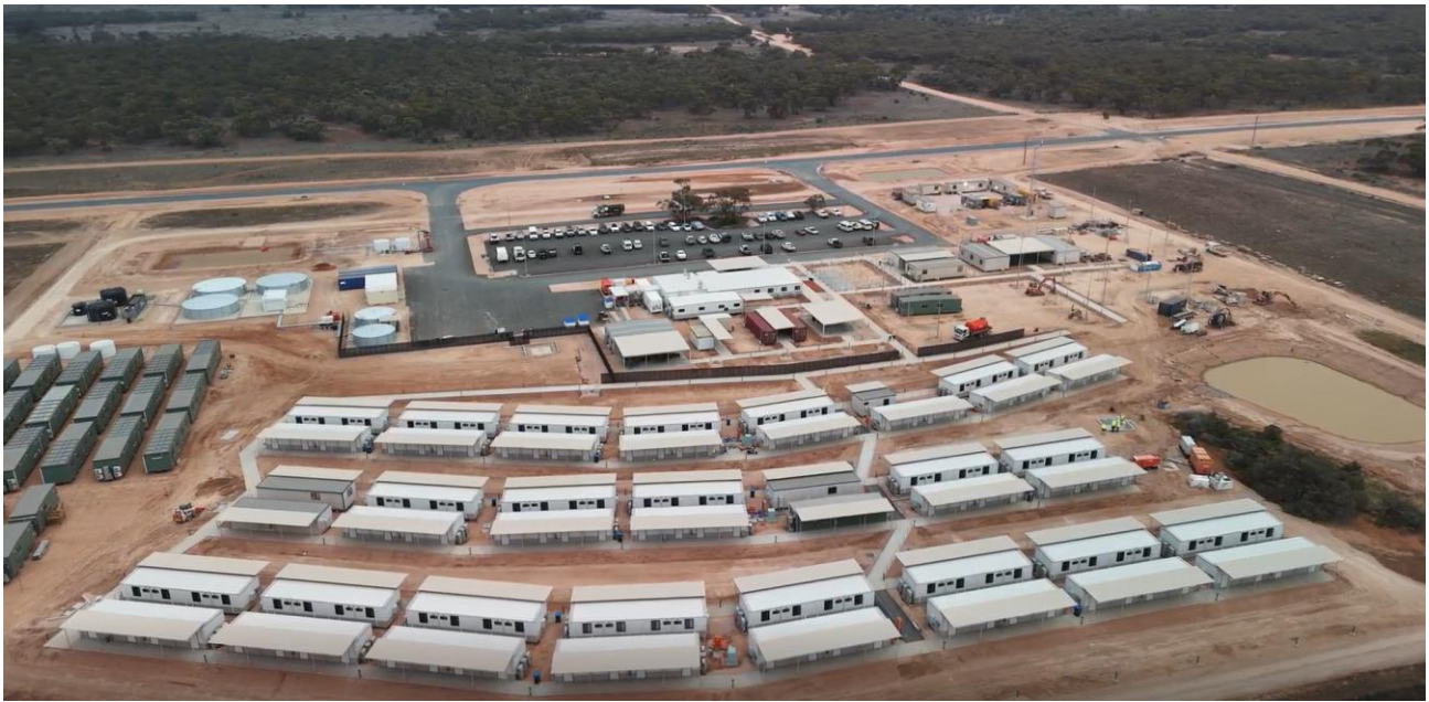
Plate 3- Construction of accommodation camp facilities
