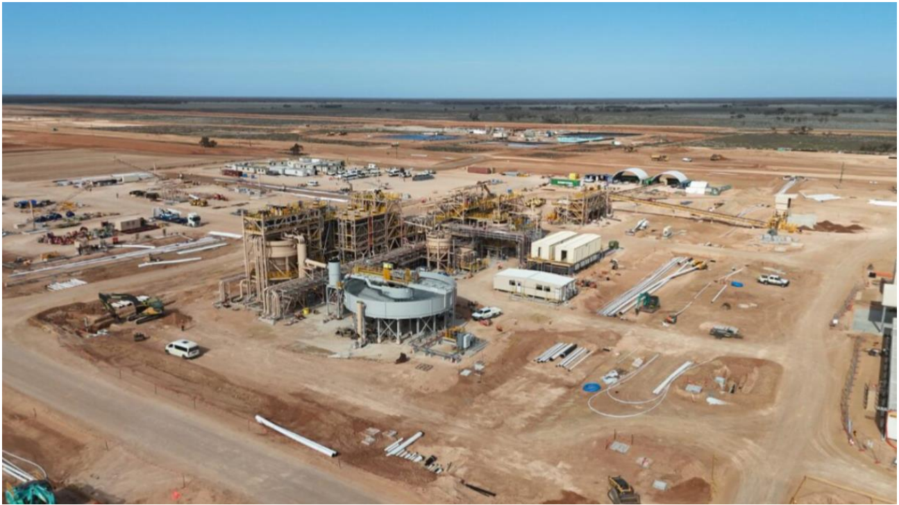
Plate 1- Wet Concentrator Plant (WCP) construction
