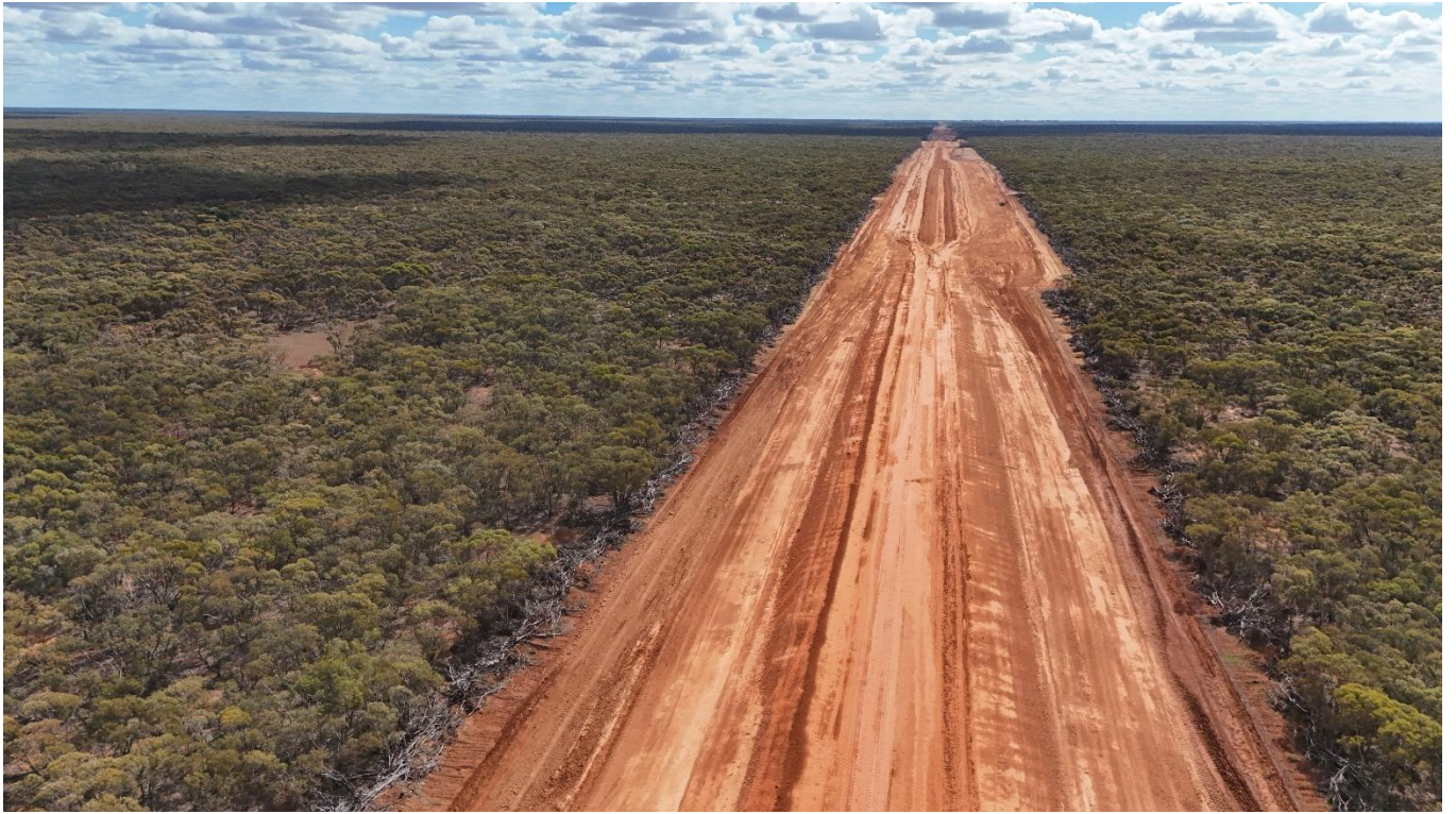
Plate 3- Mine access road construction
