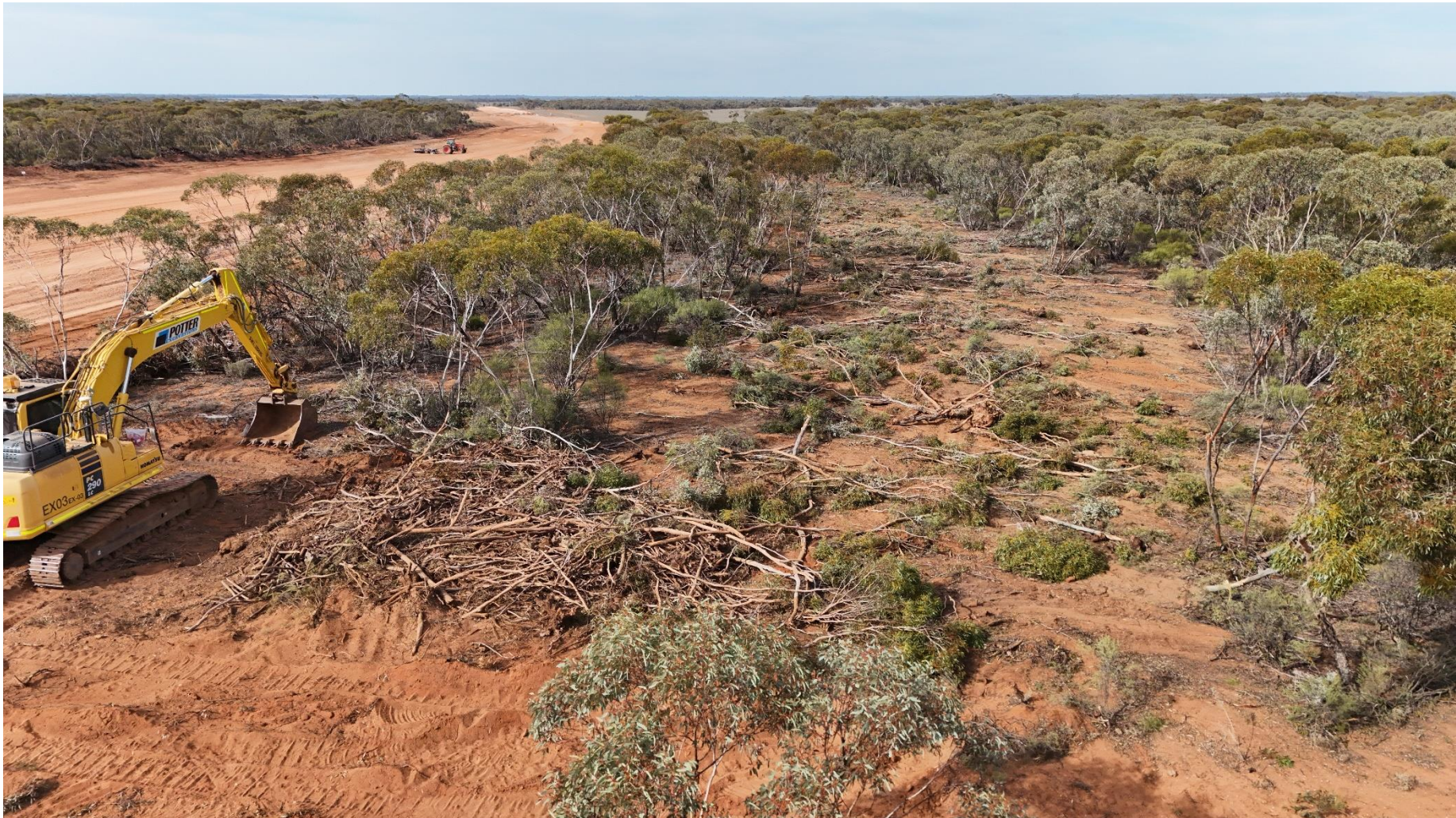
Photo 1- Mallee trees spread back over cleared area
