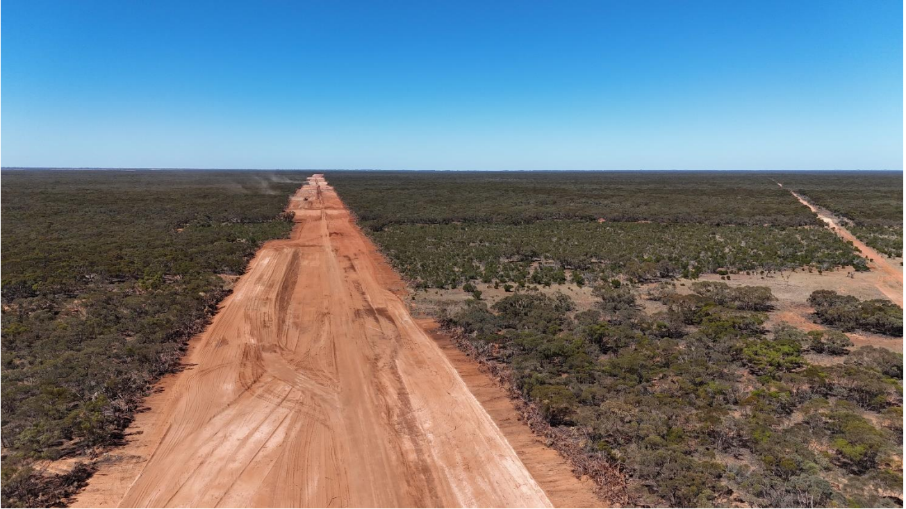
Mine access road clearing (March 2024)
