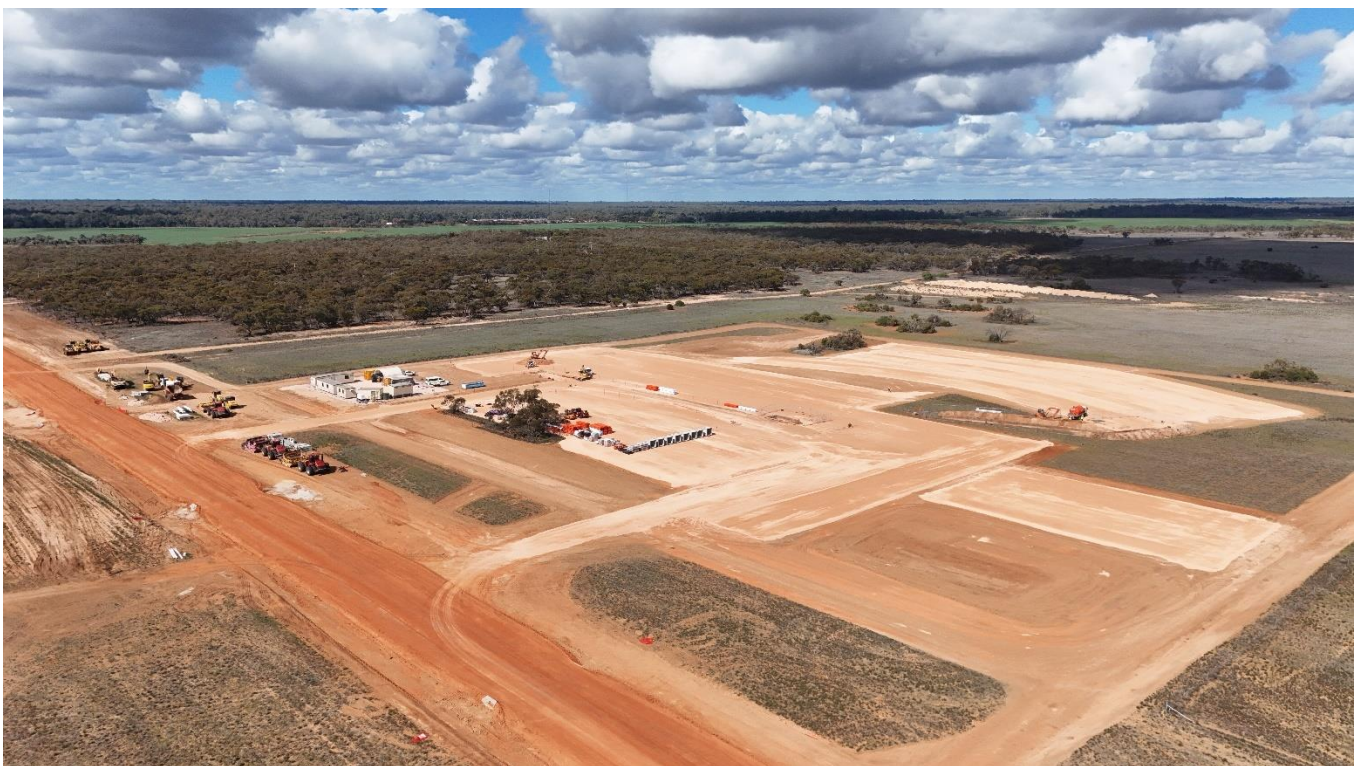
Plate 2- Accommodation village construction works
