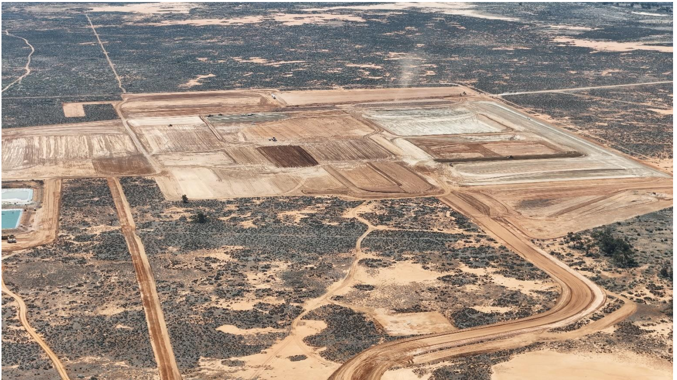
Plate 1- Processing plant area construction
